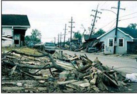
The devastation of the Lower Ninth Ward caused by Hurricane Katrina.
